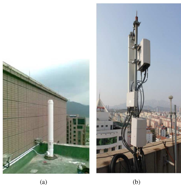
Fig. 14. Application example for the (a) proposed base station antenna and (b) ordinary plate base station antenna, respectively.
