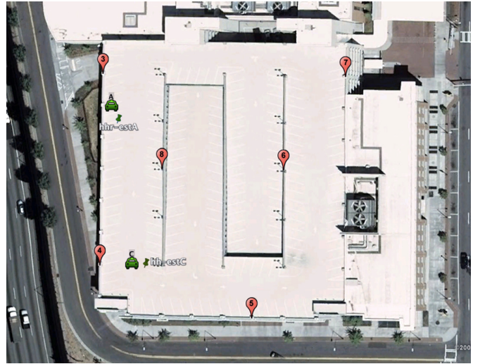
Fig. 4. The Georgia Tech hotel's parking deck rooftop
